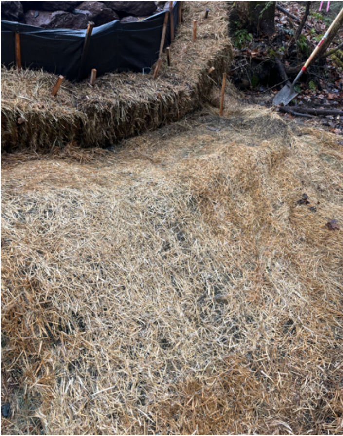
The matting was removed, stones cleaned, and erosion mat was reinstalled.
