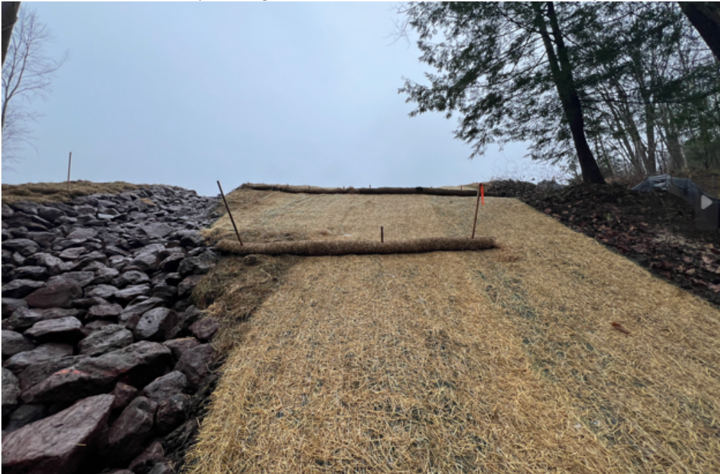
The matting was removed, stones cleaned, and erosion mat was reinstalled.
