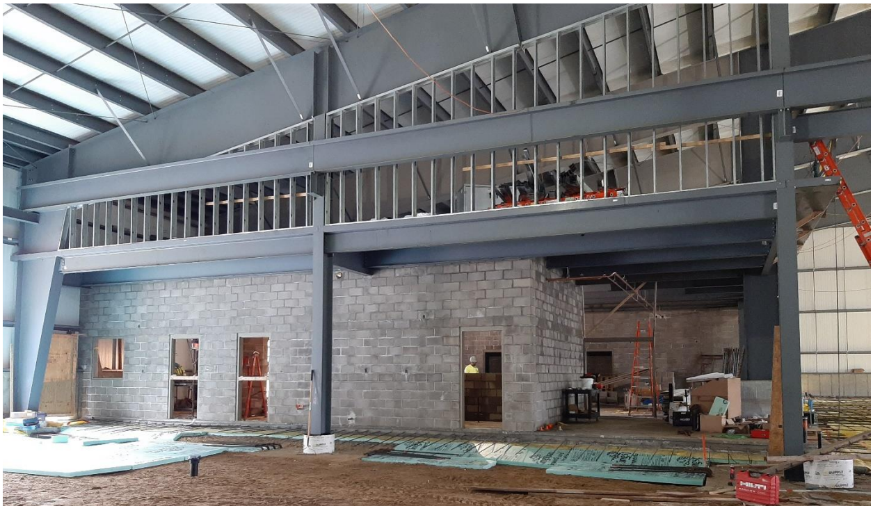
Photo 5 & 6 - Masonry Partitions at Lower Level / Maintenance Bays
